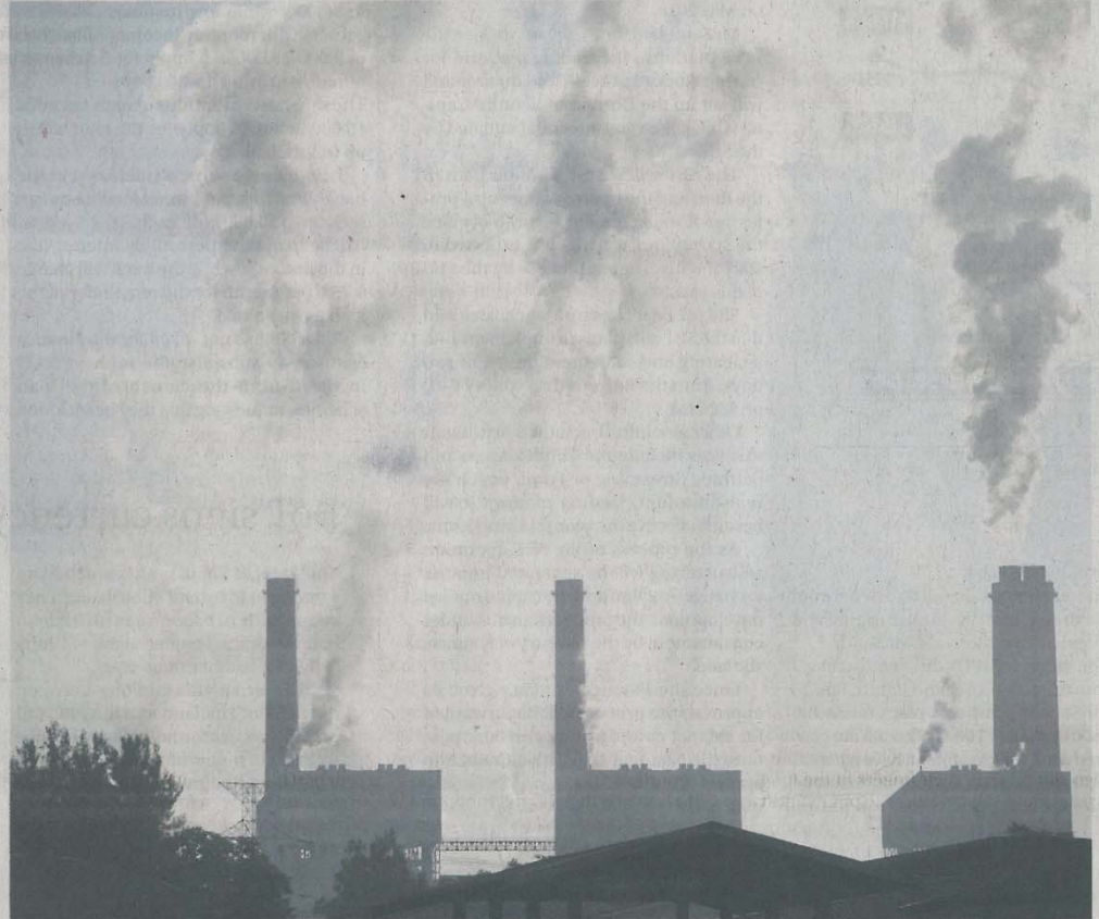
Egat's Mae Moh power plant in Lamphang. Both fossil fuels and renewable energy will be deregulated. JIRAPORN KUHAKAN
