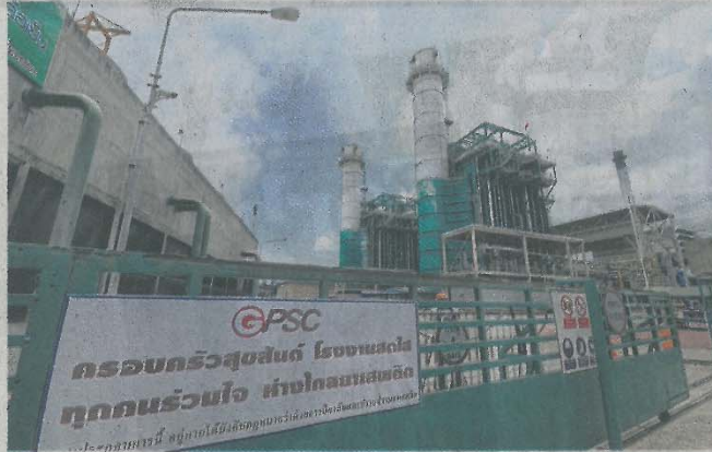
GPSC's power plant in Sri Racha. The firm is attempting to acquire Glow Energy.
