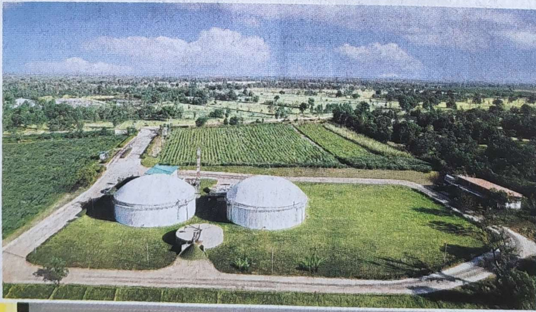
A 1.2-megawatt biogas-fired power plant in Ubon Ratchathani's Sawang Wirawong district.
